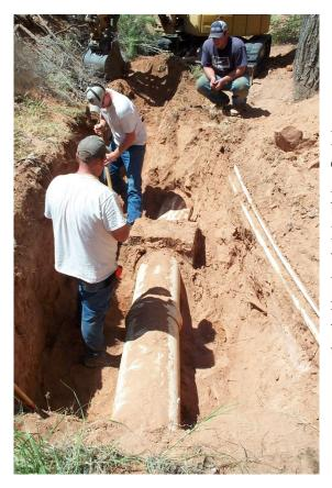
Digging into the line, we soon discovered a cement block that we did not know existed. Apparently, sometime in the past, there had been a leak at this point in the line. Most like due to trying to bend the line around a tree. To stop the leak, duct tape and cement was used to stop the leak. That kind of repair does not hold and with a tree right there looking for water, roots soon entered the line and began to expand.
