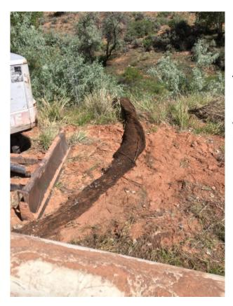
A root plug that had to be at least 15' long was found inside the 15" diameter pipe. This was a large root plug. The water flow was much improved after its removal.
