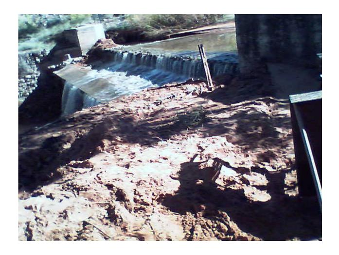
A lot of sand was deposited inside and on top of the sand box for Center Ditch 2. It took several days and a large water truck to clean the sand off and out of the system. Shareholders often do not know what the water master deals with behind the scenes to keep the water flowing in the irrigation system.
