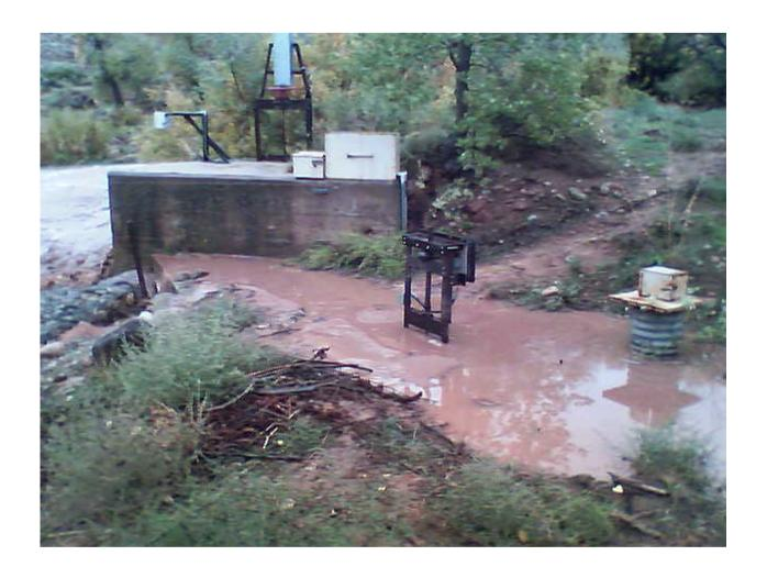
Water flowed around and over the sand box of Center Ditch 2 and it filled the sand box with sand, it plugged the exit pipe that allows water to go back into the creek and it put a fair amount of sand into the main irrigation pipeline that had to eventually be flushed out.
