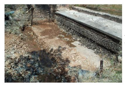
Then a ditch was dug to create an end footer to anchor the apron.
