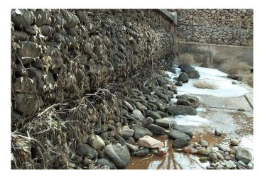
In this picture you can see how the gabions were shedding rocks. The wires holding the gabions together were breaking in my locations.
