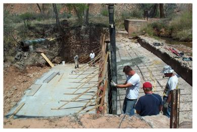
A massive wood wall was built to hold the cement pour of the face of the dam.
