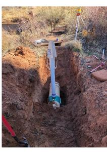
his properly. In the future if the line for some reason sprung a serious leak in this area, it could be pulled out of the sleeve, repaired, and reinserted.
