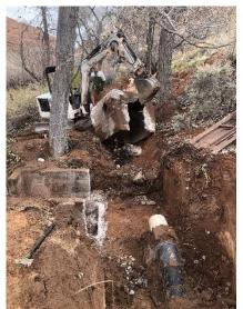
We now had to reverse the machine and weld on a few more lengths in the other direction to get back to the PIP pipe flange. This was a little challenging in the tight area we were working. To connect the PIP pipe to the HDPE pipe, flanges are used to bolt the pipe together.
